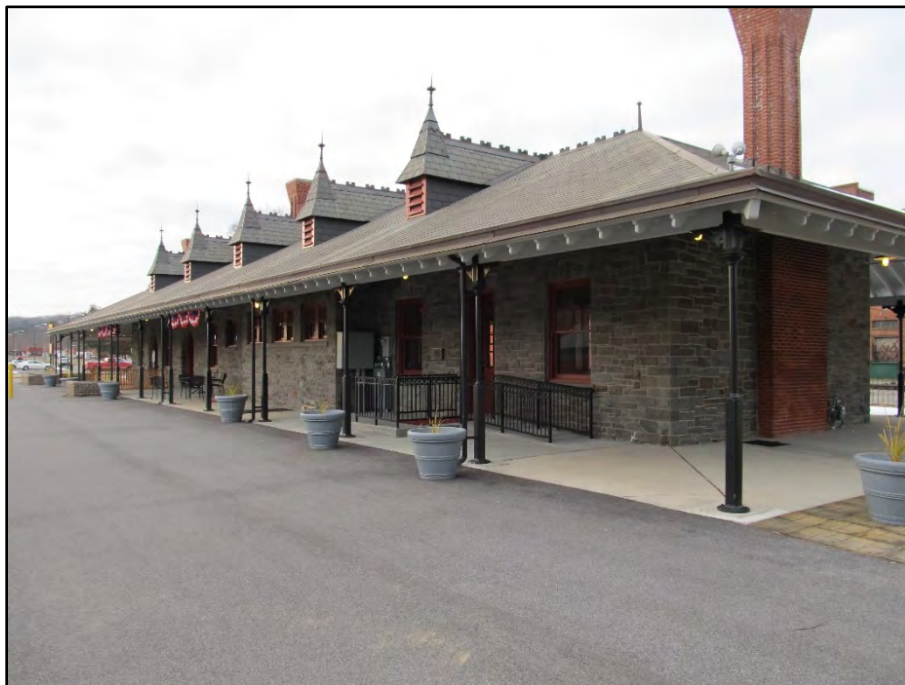
The reconstructed train station was completed in June 2011.
