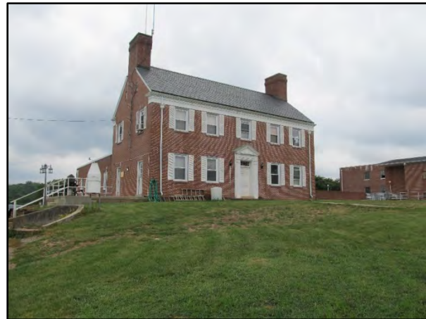
Water Filtration Plant on Randolph Avenue.
